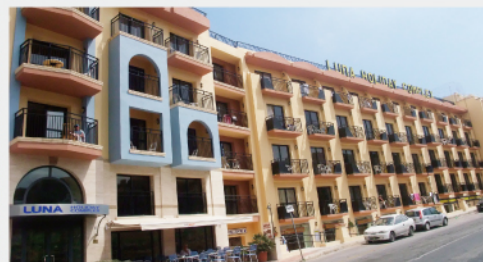
Luna Holiday Complex Water-cooled Screw Chiller Malta
